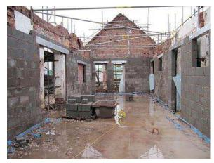
The beginnings of our Butchery and Farm Shop. Here you can see the recycled aggregate block we used to support the upper floor and roof.
