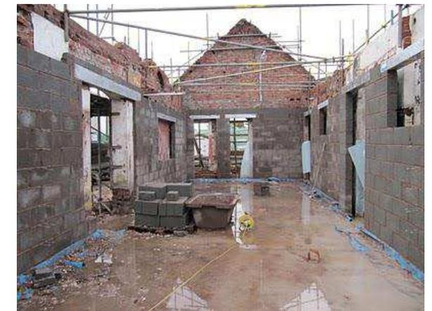
The beginnings of our Butchery and Farm Shop. Here you can see the recycled aggregate block we used to support the upper floor and roof.
